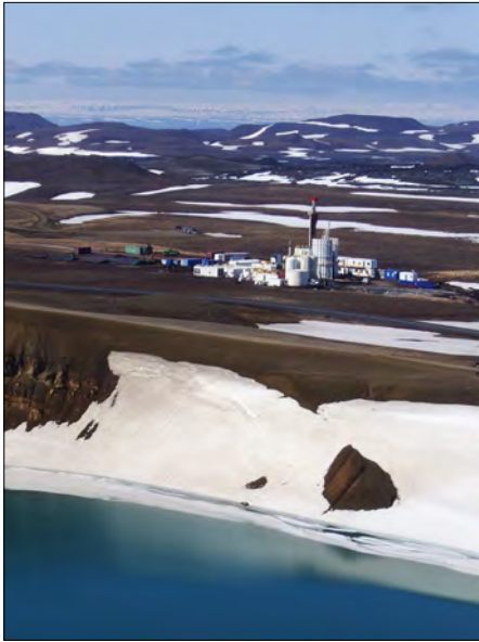
Well IDDP-1, the first deep well of the Iceland Deep Drilling Project (IDDP), penetrated rhyolitic magma at a depth of 2104 m in the Káfla Geothermal Field in northern Iceland (see map). Pictured is the rig (now removed) used to drill the well. The well overlooks Viti, an explosion crater formed in an eruption in 1724. Photo by G. Ó. Friðleifsson, July/Aug. 2009
