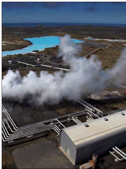
The Reykjanes Geothermal Power Plant is on the Reykjanes peninsula in southwestern Iceland. To operate the single-flash power plant, brine with the salinity of seawater is extracted from 11 production wells drilled 2700 m deep into a reservoir where the temperatures range from 280 to 316° C.
