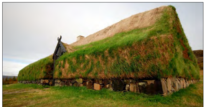
Stöng, a reconstructed Viking longhouse in the Tjórásadalur Valley, east of Laugarvatn. Such longhouses were the farm centers for Viking chieftains in the Middle Ages and were used to store food. This replica was rebuilt as closely as possible to the original longhouse specifications. You can see portions of the basic wooden frame, a stone base, and the turf walls and roof. The original building was buried in volcanic ash during an eruption of Mount Hekla in 1104. The site is open to the public. Courtesy of The Commonwealth Farm, www.thjodveldisbaer.is
