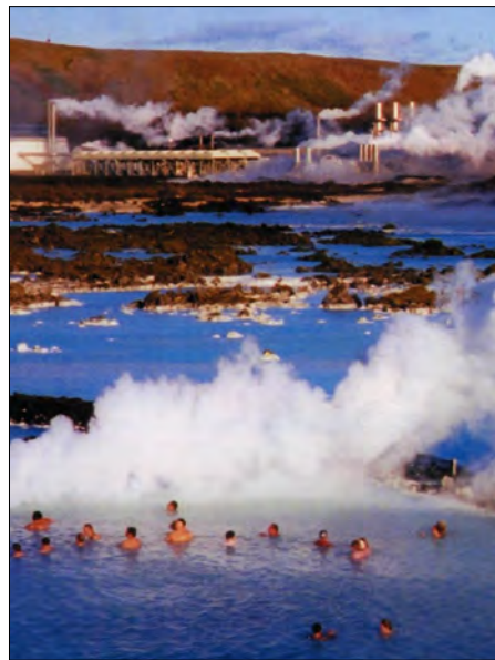
The Svartsengi Power Plant, in the Sudurnes area, is the world's first geothermal power plant to both generate electrical power (361 MWe and 125 MWt) and produce hot water for district heating. It also provides water to the Blue Lagoon, pictured here, a bathing resort attracting tourists worldwide. Photo by John W. Lund, March/April 2006
