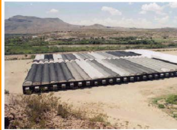
Masson Greenhouses at Radium Springs – Source of photo: Geo-Heat Center at the Oregon Institute of Technology (OIT) – GHC Bulletin, December 2002
